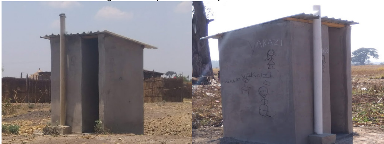
Figure 8: Small Blair toilets servicing the entire Lydiate community
