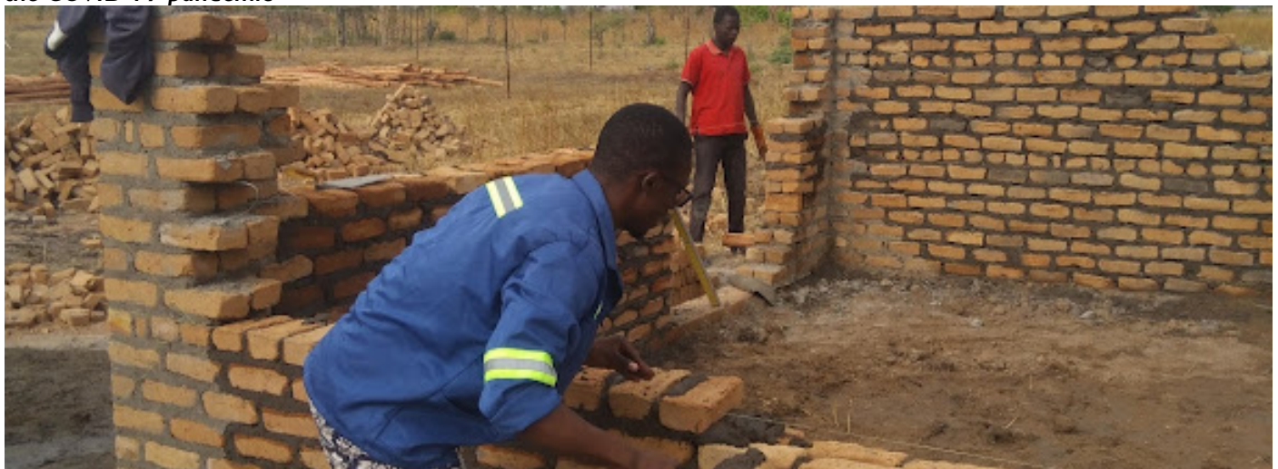
Figure 4: The researcher working on a building project with some migrants from Lydiate informal settlement before the COVID-19 pandemic
